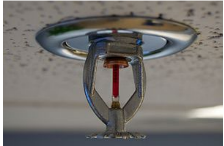
Active Fire Protection e.g. Roof Sprinkler System Image source: Wikipedia
