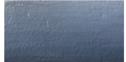
An example of what might be considered a Basic finish (viewed from 2m)
